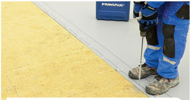
The flat roof insulation system involves insulating new or existing roof surfaces. The thermal insulation material (mineral wool, PIR/PUR, EPS) together with the membrane (EPDM, PVC, TPO/FTO, bituminous) is fixed to the substrate using mechanical connectors. The whole is covered with a thermally welded membrane (PVC, EPDM, TPO/FTO, bitumius), which protects against changing atmospheric conditions and mechanical damage during everyday use.
